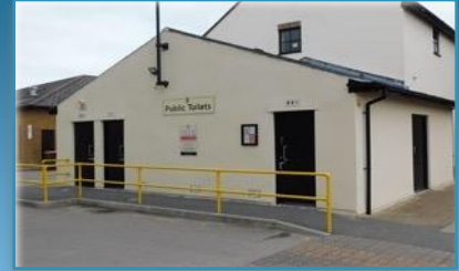
Borough fields Toilets (£10,734)
